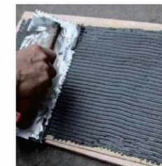
Apply adhesive mortar on the back of the tile.
