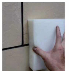
Wipe off remaining dust and residue with a sponge.
