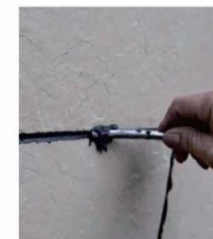
When the grout is half dry, smooth the seams with a jointing tool.
