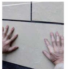
Move the tile up and down to adjust the joint width, then press firmly with a rubber board.
