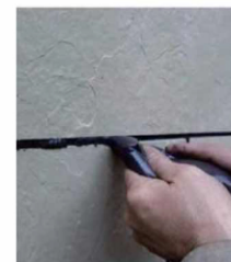
Fill the joints with grout using a plastic rod bag, or apply silicone sealant.
