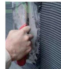
Apply adhesive mortar on the wall surface.
