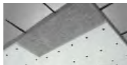
Fire Rating Ceiling System
